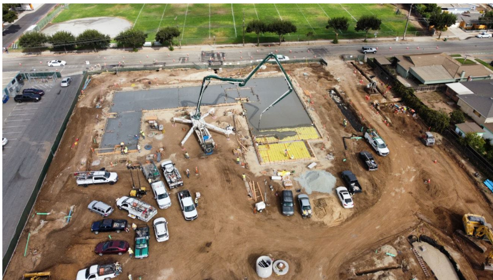
Ariel view of Building A slab pour.
