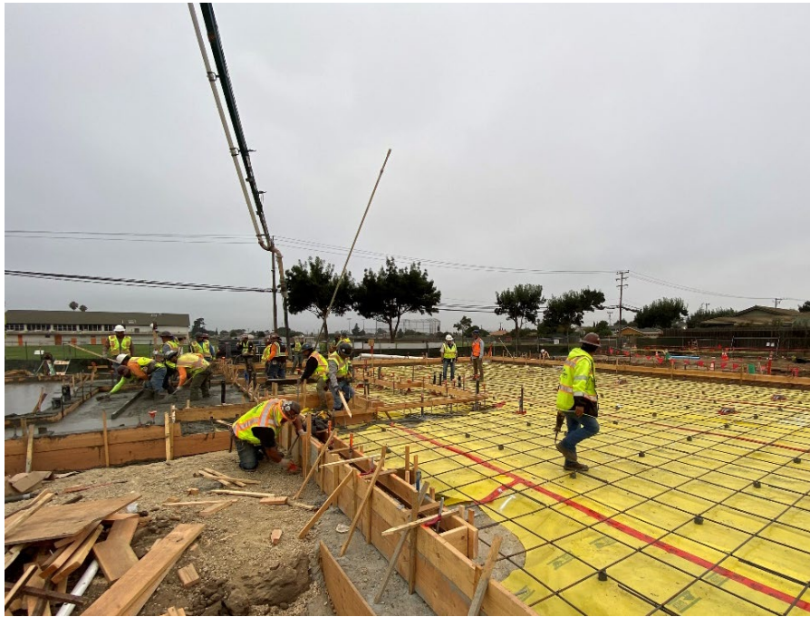
Building A pad reinforcement and concrete pour.
