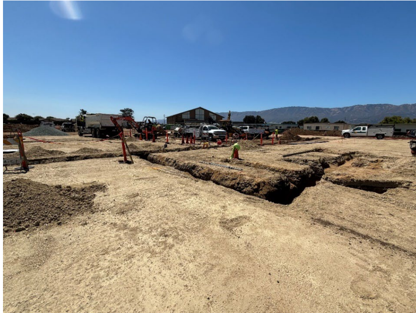
Building A under slab plumbing utility trenches.
