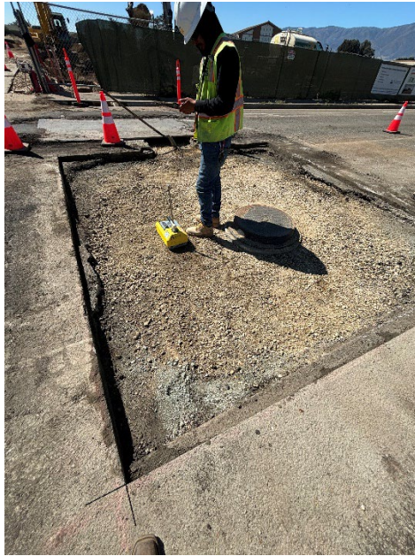
New Sanitary Sewer Manhole at Fifth Street.
