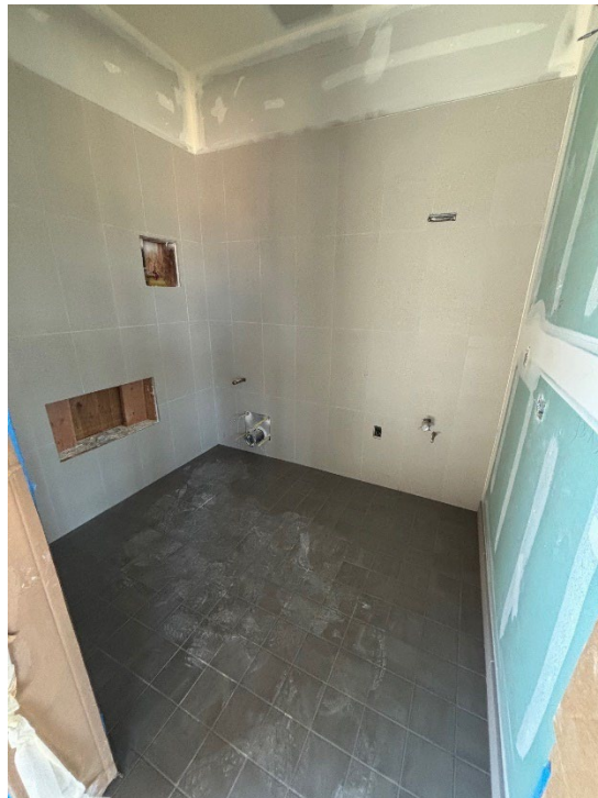
Ceramic tile progress installation at Family Restroom A131 (May 2025).
