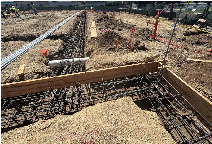
Building A Footing Reinforcement.
