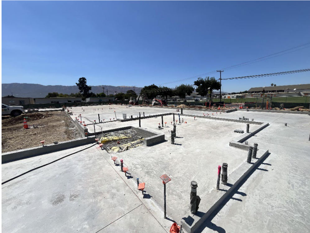
Finished Slab on Grade (Building A).
