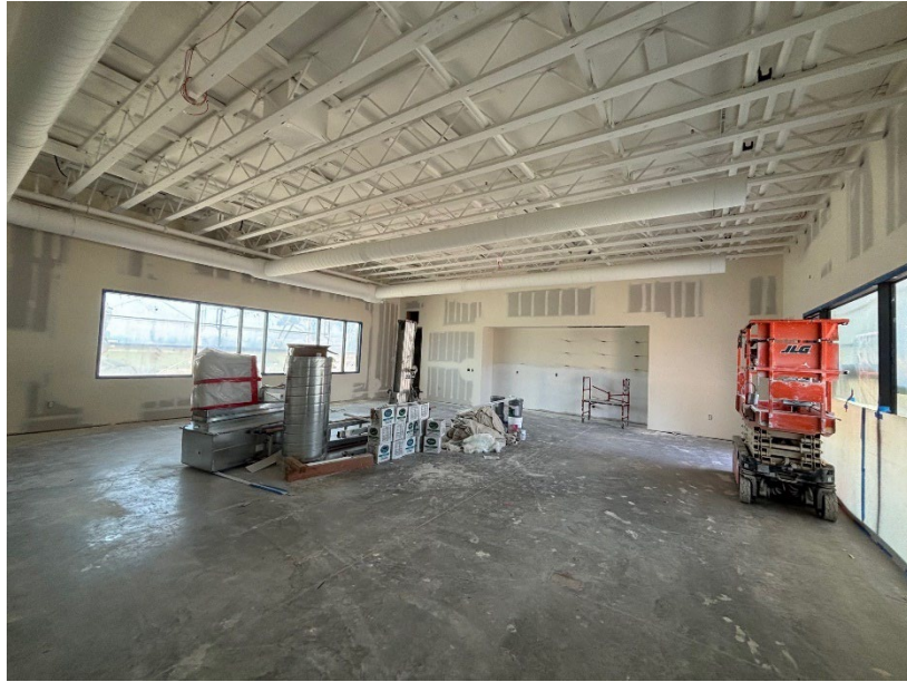
Interior drywall taping and finish at Teen Innovation Center (May 2025).
