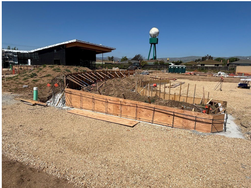
Amphitheater seatwall formwork and reinforcement (April 2025).
