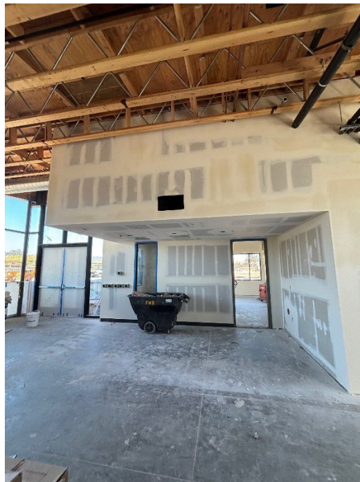
Interior drywall taping and finish at Library (May 2025).
