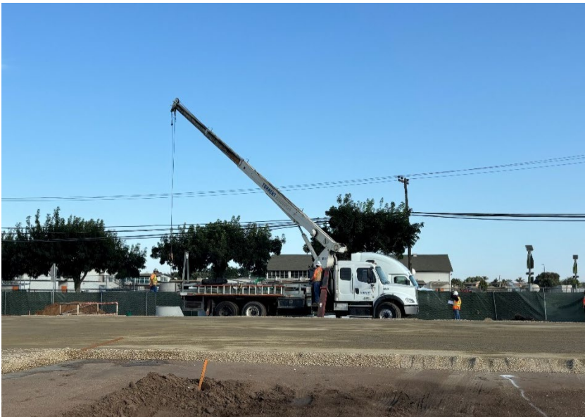
Installation of Dry Well (stormwater management).
