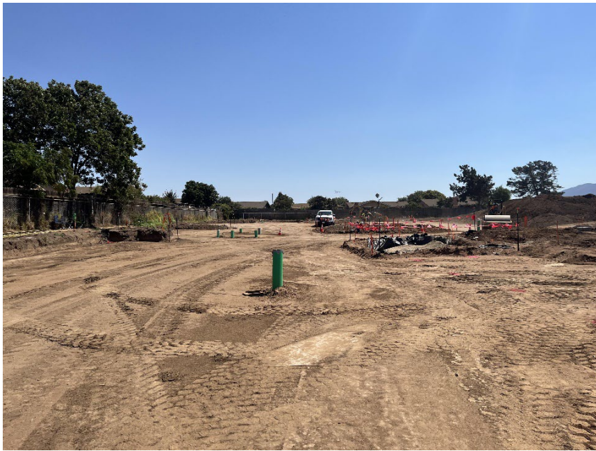
Site Grading (Driveway and Parking Lot).
