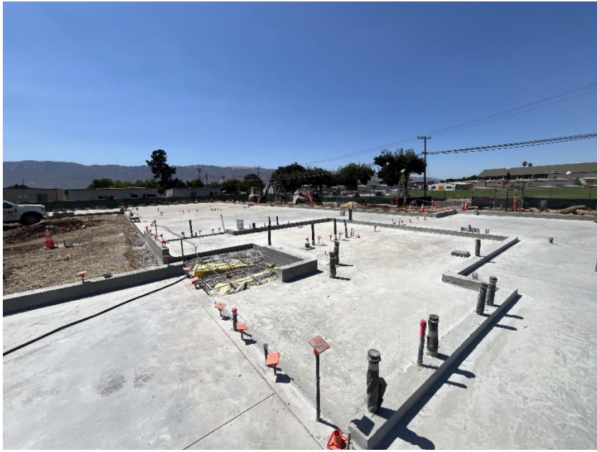
Finished Slab on Grade (Building A).
