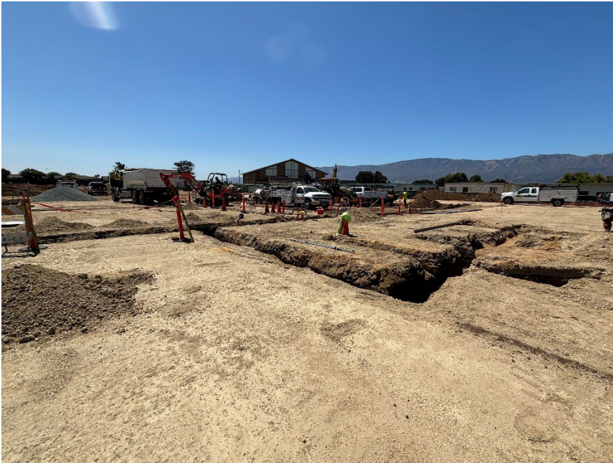
Building A under slab plumbing utility trenches.
