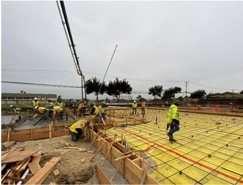
Building A pad reinforcement and concrete Pour.
