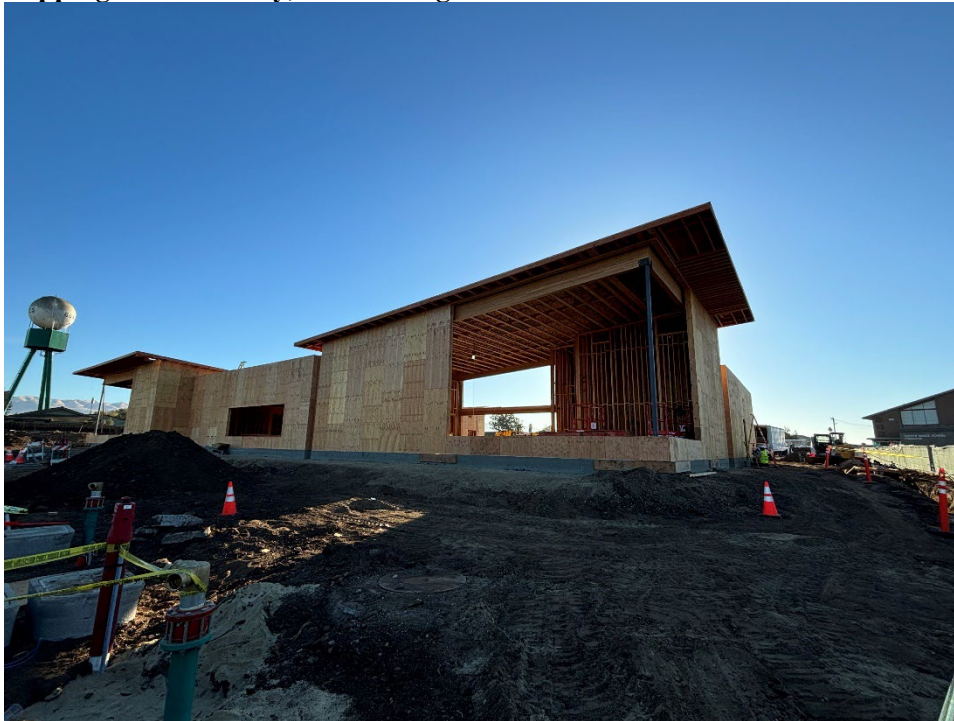
Northwest exterior elevation of Building A.
