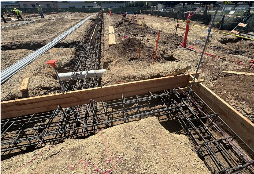
Building A Footing Reinforcement.
