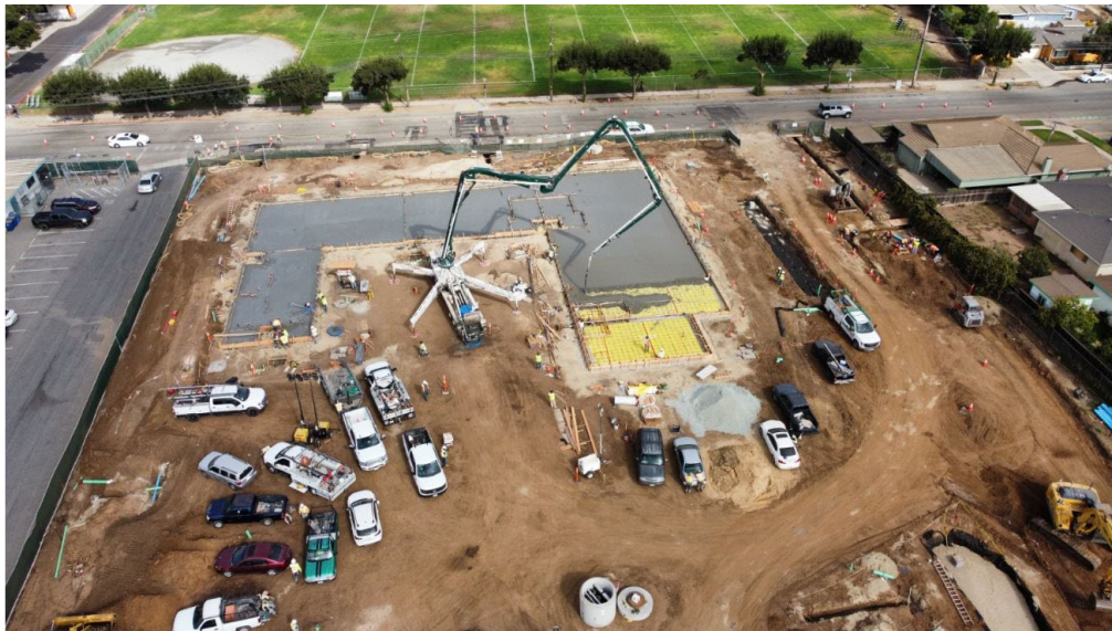
Ariel view of Building A slab pour.
