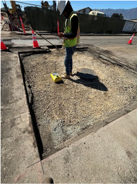
New Manhole Installation at Fifth Street (progress installation).
