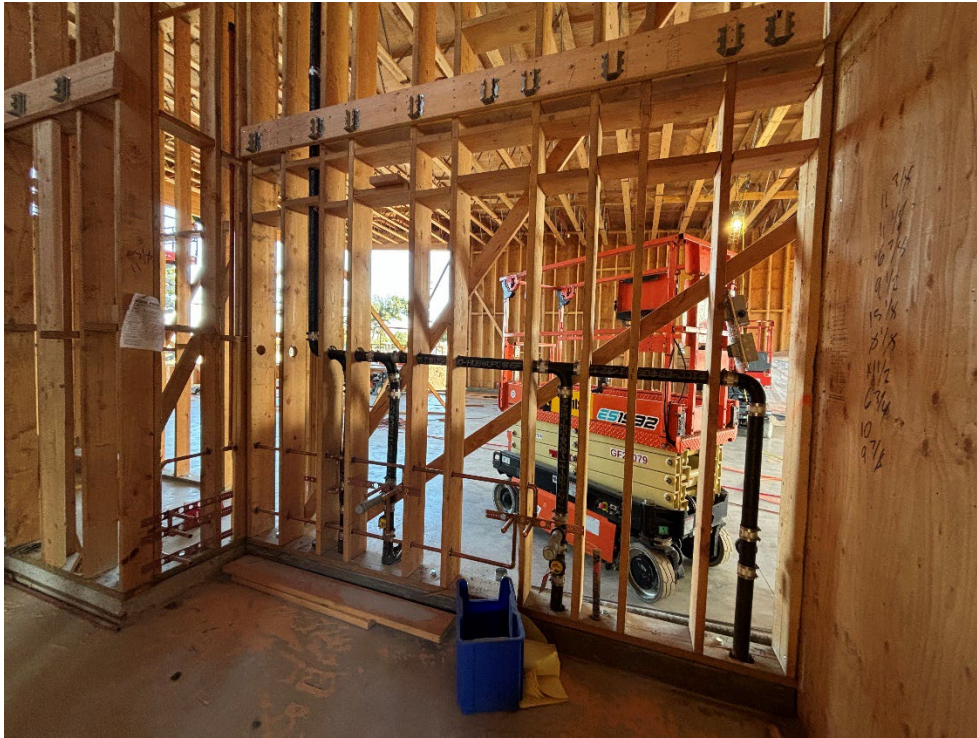
In-wall plumbing rough-in progress.
